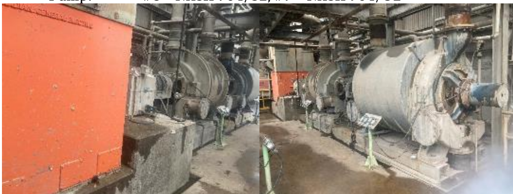
1 st Press Top/Bot Press Felt #10 and Trivac #11 Vacuum Pumps
