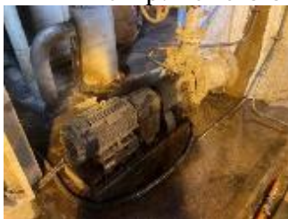
High Pressure Fresh Water Shower Pump
