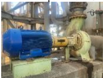
Recycle Dilution Pump
