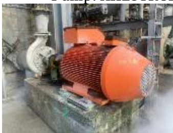
Clear White Water Pump Motor: POPE, D315M, 415V/75kW/6P Pump: AHLSTROM APP51-300, 317l/s, 16.6m
